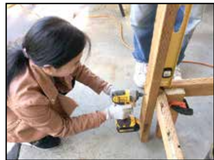
Ve Bui builds the frame.
