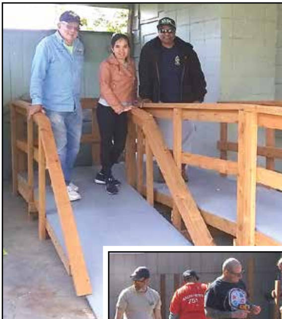
Above: Jim Hutchins, Ve Bui, and Princie Stewart on the finished Bellevue ramp.
