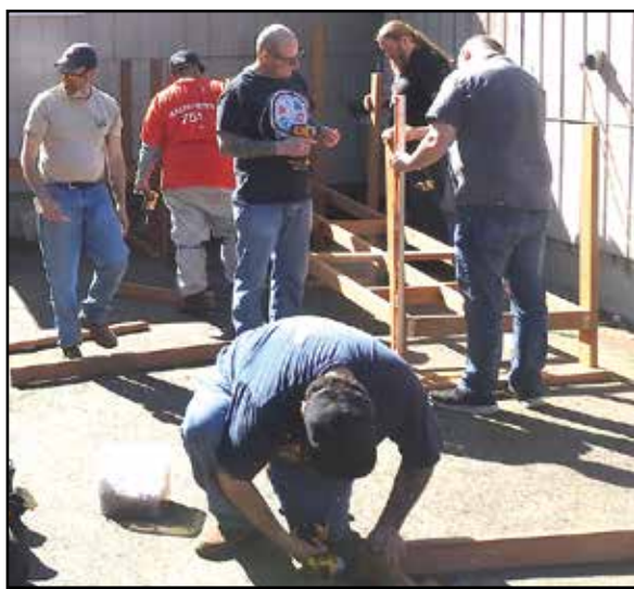
Above: volunteers building the ramp for family of a member in Arlington.
